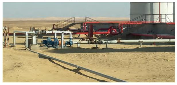
Figure All.4: Shipping Pumps at El Salmiya Oil Station
