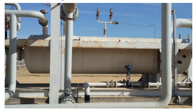
Figure All.6: FWKO Vessel and its Valves
