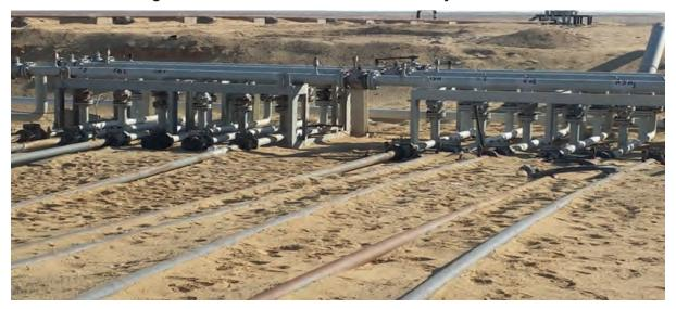
Figure All.2: Production Manifold at El Salmiya Oil Station
