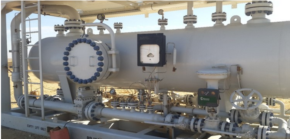
Figure AIV.3: 3-Phase Separator
