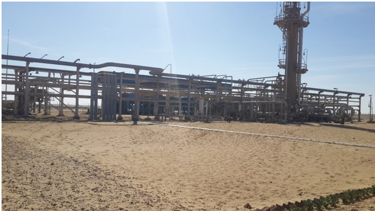
Figure AIV.5: General View of Gas Facility
